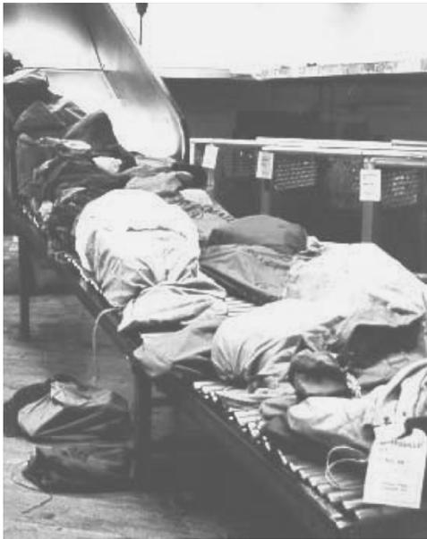
Fig. 2. In some distribution centers, the mail sacks travel down a narrow chute and drop onto conveyor rollers, and are then manually moved directly onto rolling carts based on destination.
